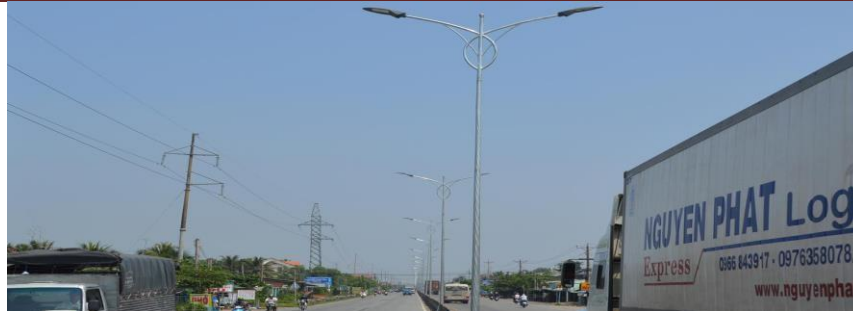
Fig. 1. Lighting systems on NH1
